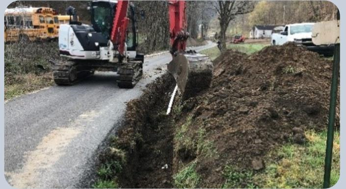
The Hindman Waterline Extensions project was funded by a \$625,192 CDBG grant and \$600,000 ARC grant to provide service to 102 households. The project constructed a total of 21,949 linear feet of new waterline and installed a new pump station.
