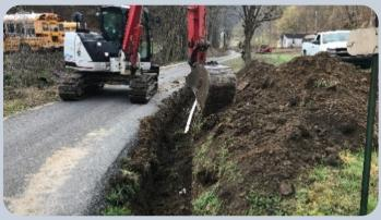
The Hindman Waterline Extensions project was funded by a \$625,192 CDBG grant and \$600,000 ARC grant to provide service to 102 households. The project constructed a total of 21,949 linear feet of new waterline and installed a new pump station.
