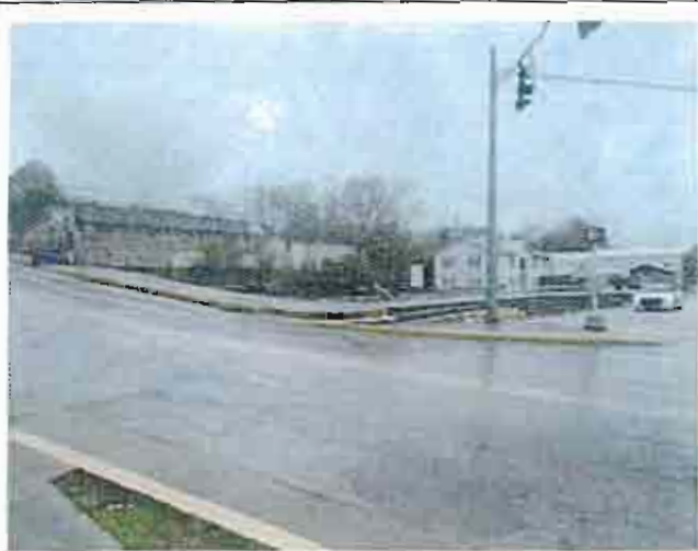
Stacey Hotel burned and is now a vacant lot.
