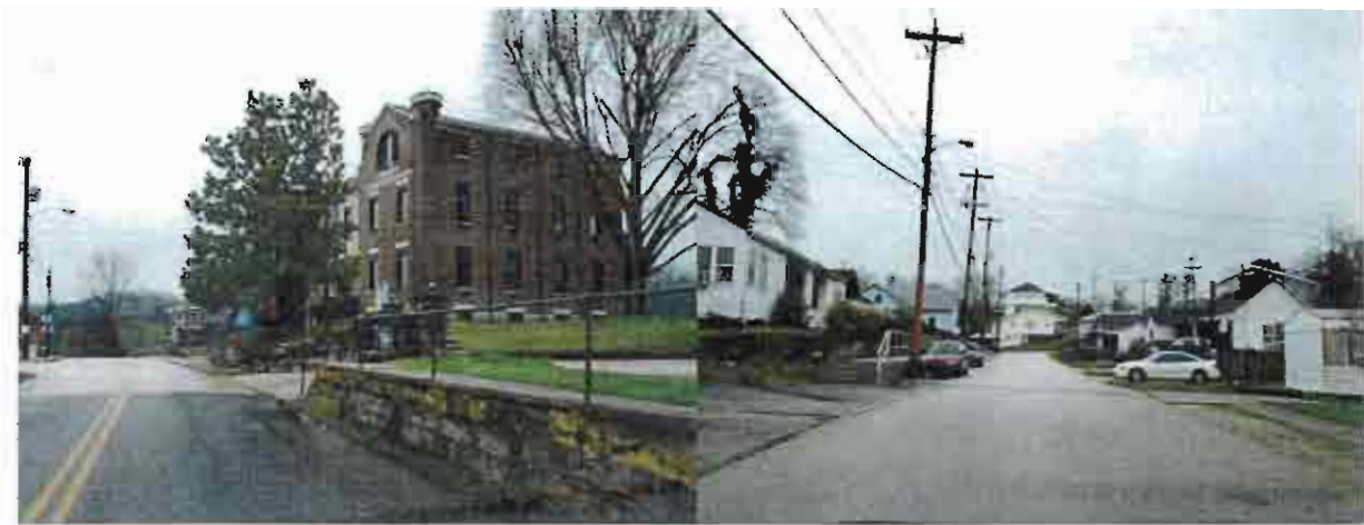
Highland Avenue (cont.)
