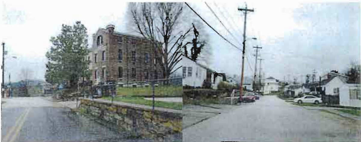
Highland Avenue (cont.)
