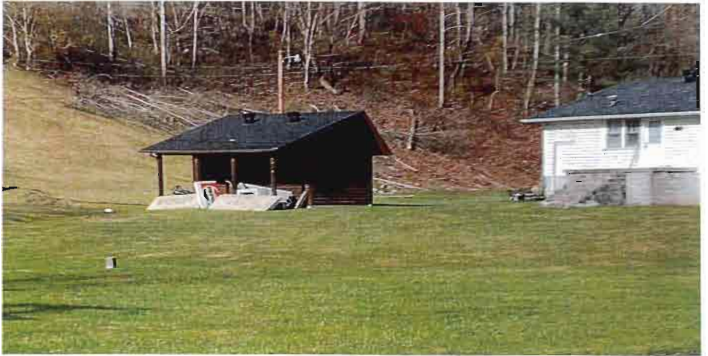
Triggers Lift Station – East View
