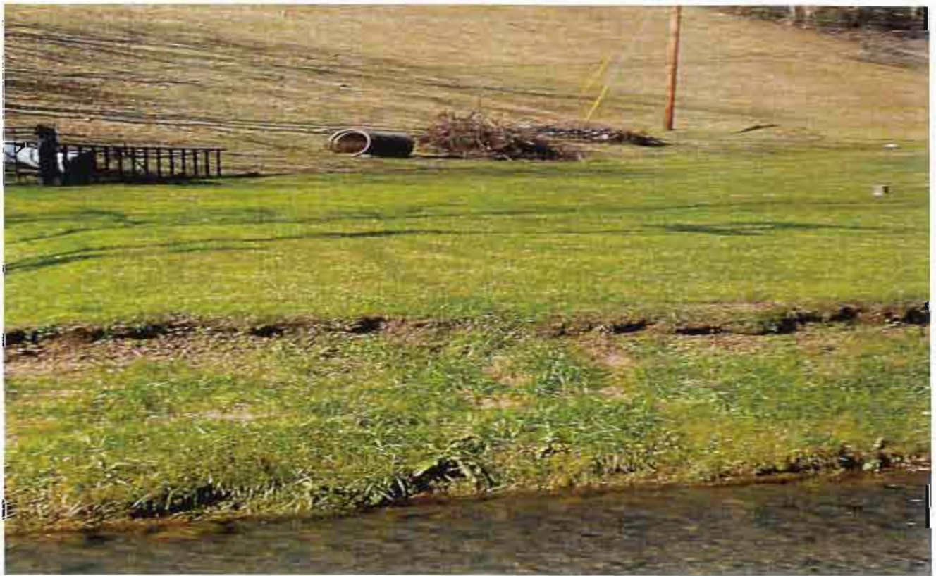
Triggers Lift Station – West View
