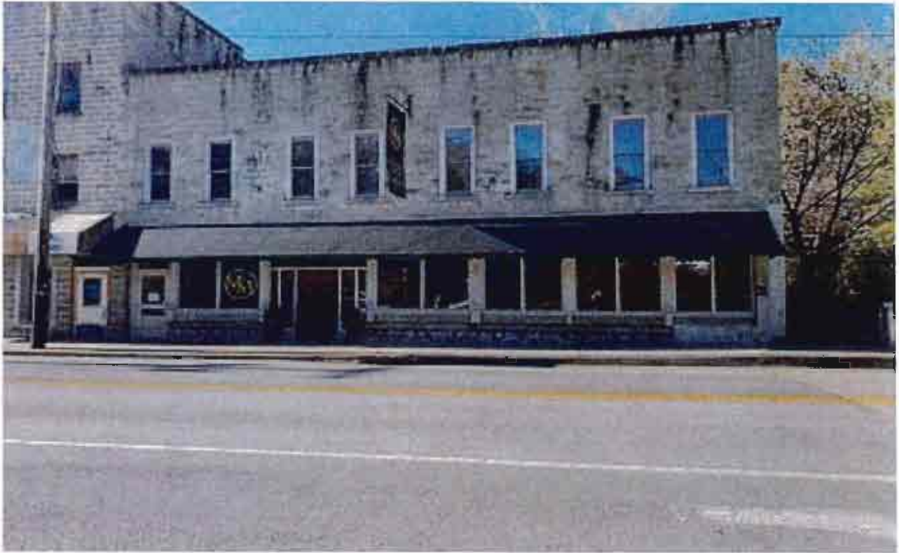
254 South HWY 160 Hindman, KY. – Front View
