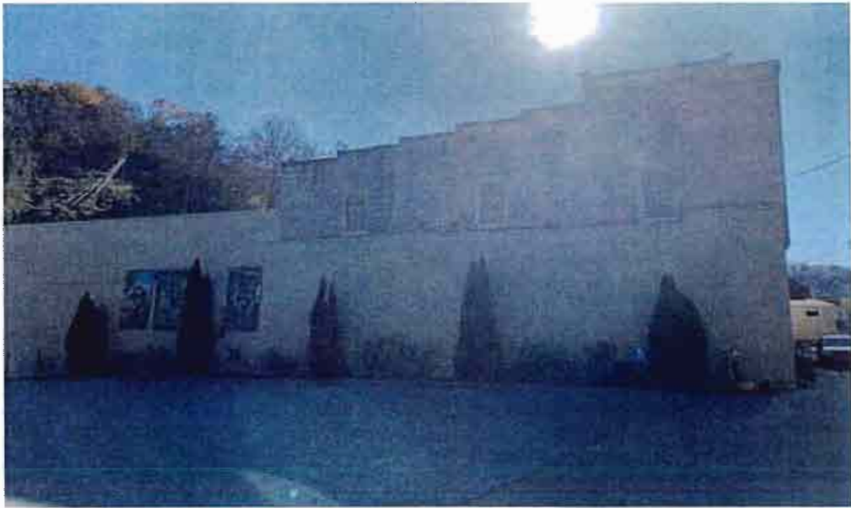
Front View of Building on SE Side of Main Street
