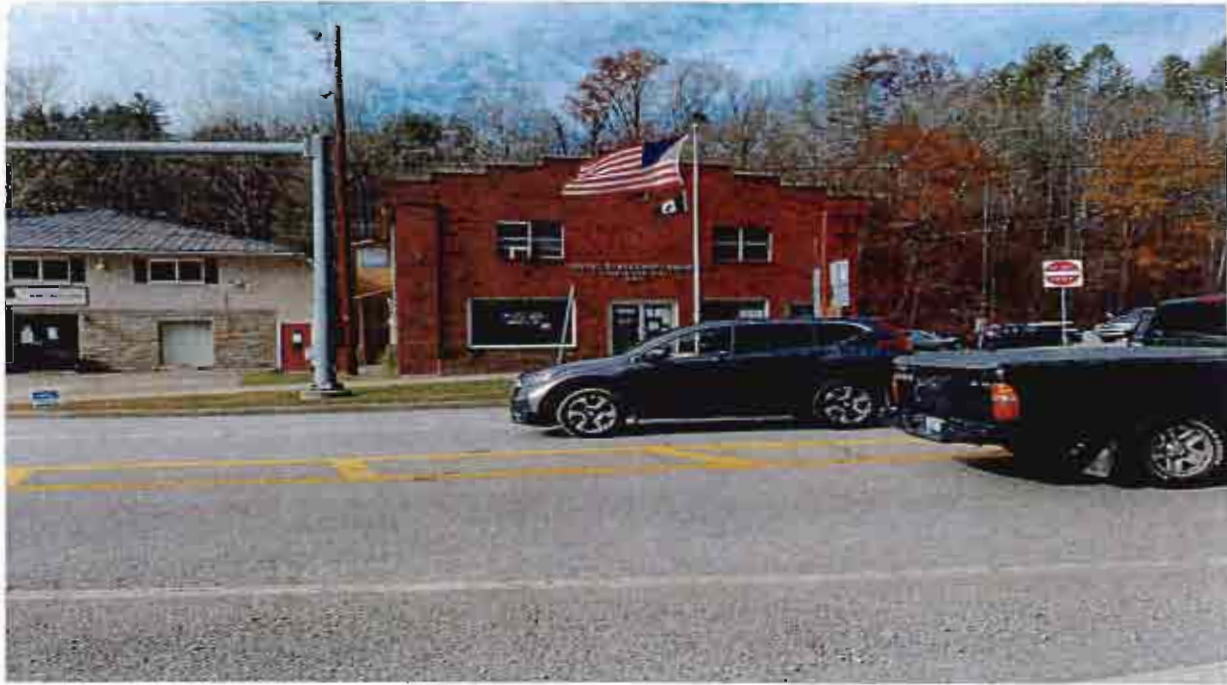
27 East Main Street Hindman, KY – Aerial View
