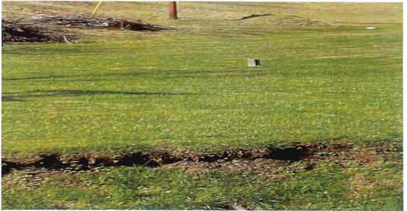
Triggers Lift Station – South View
